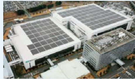
PV panels installed at Koshi Plant
