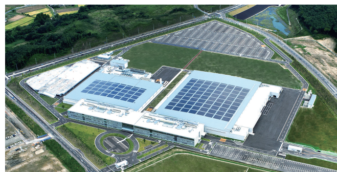
Tokyo Electron Miyagi Limited Head Office
