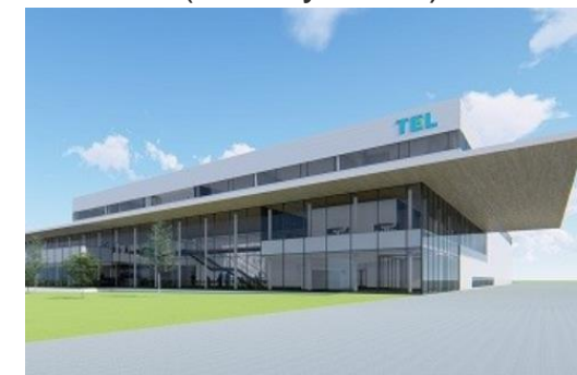
Kurokawa-gun, Miyagi Prefecture: approx. ¥7.0B construction cost (Completion scheduled for September 2021)
