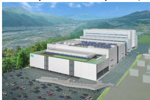
Nirasaki City, Yamanashi Prefecture: approx. ¥13.0B construction cost (Began operation in August 2020)
