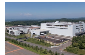
Tokyo Electron Technology Solutions Tohoku Office Production Building Began operations in July 2020
